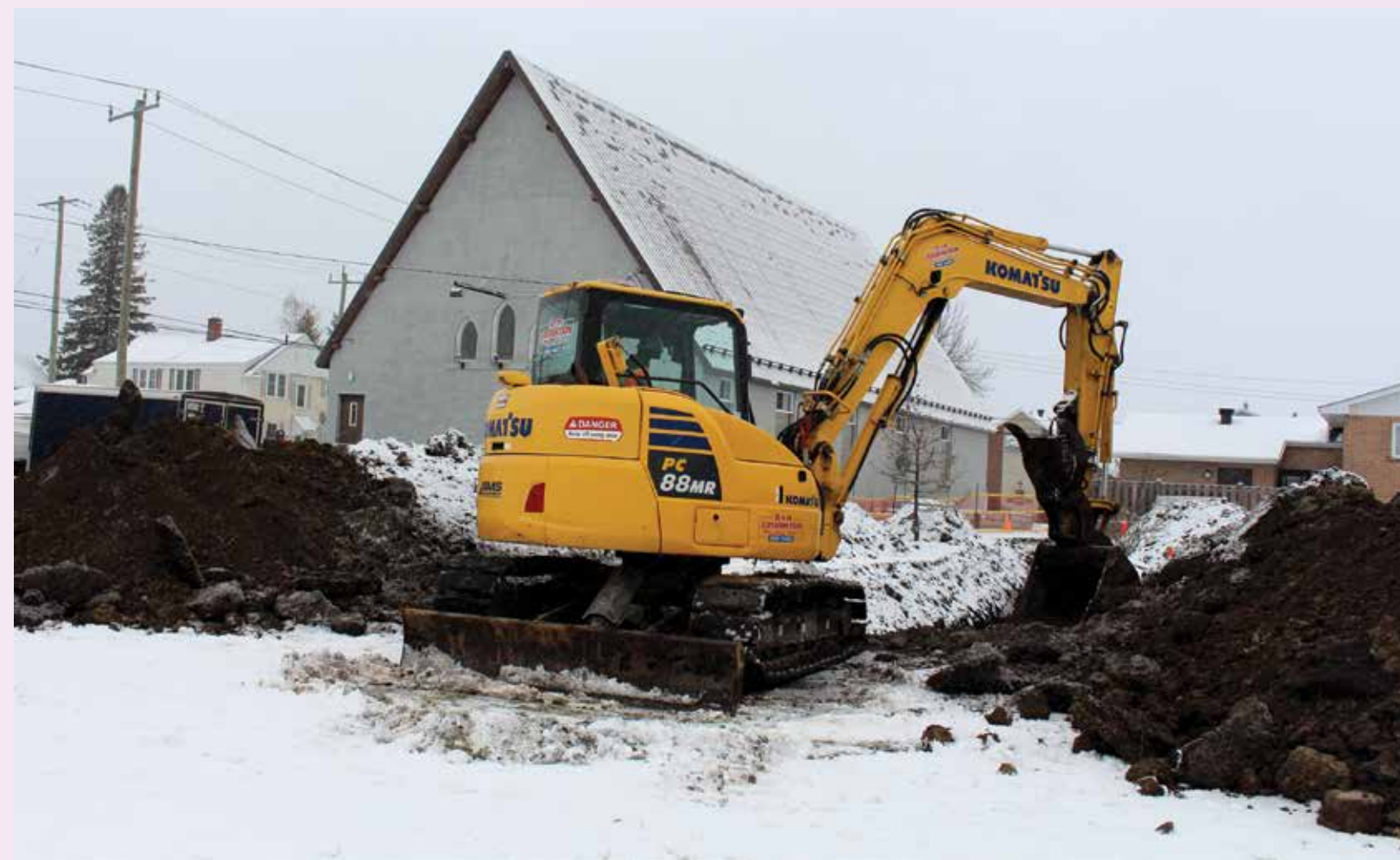
Contractors managed to dig an 8 ft. trench to connect the rectory at St. Paul's in South Porcupine to the City of Timmins' water line - for the first time since the rectory was built in 1984! Dean Valerie Isaac and her husband Ron can now have all the tea that they want.
